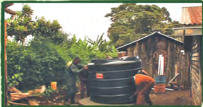
Water tank on concrete base
