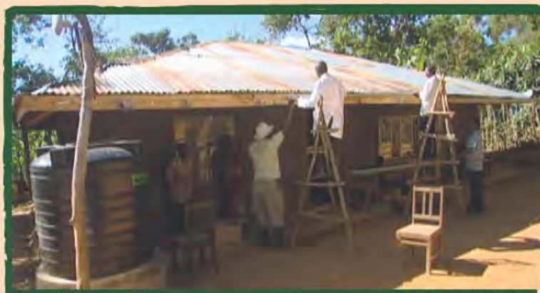
Water storage tank and guttering
