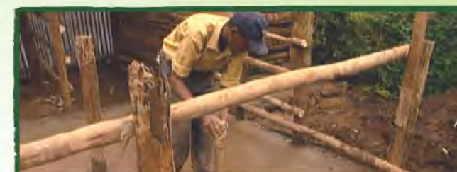
Concrete floors being made
