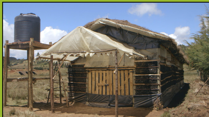
The charcoal is always kept wet by water from a tank. Water evaporates from the charcoal which takes heat from inside the store. The store is therefore kept very cold.
