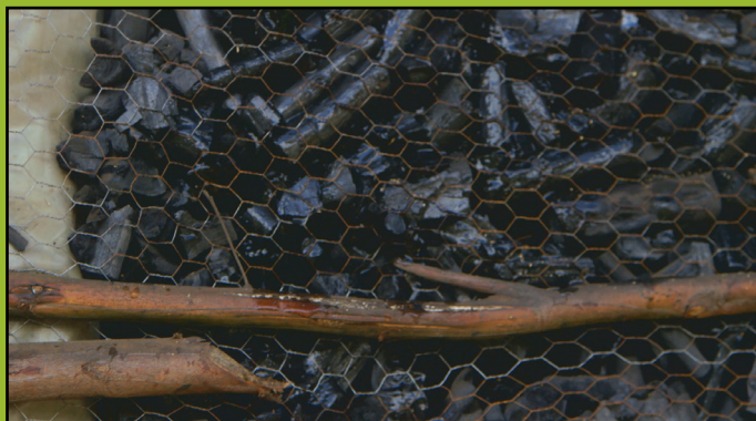
The open walls are made of mesh wire packed with charcoal.
