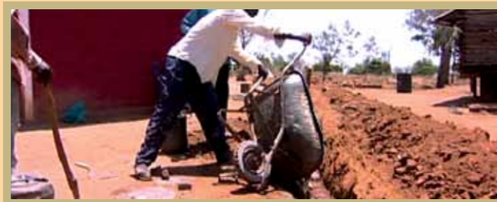
Cement pouring into the guttering
